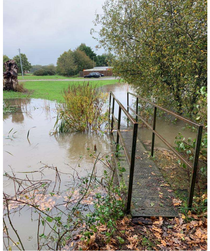
Footbridge to west of Oakendene Lake
