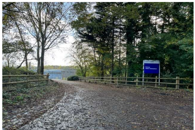
National Grid Substation, below ground level
