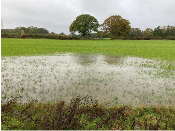
Southern end of Proposed Substation Site from the south
